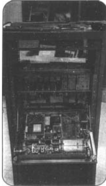
Photo D. A GE Mastr II 800-MHz repeater. This can also be modified to work on 902 MHz, but takes a different set of mods than The Exec II.
